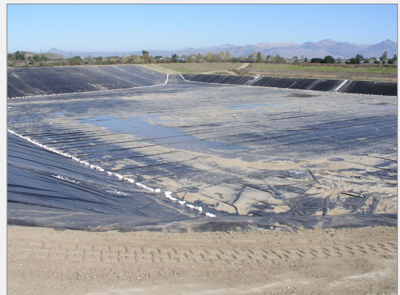
Completed pond ready for water
