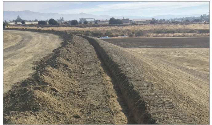
Anchor trench at top of pond to hold liner in place
