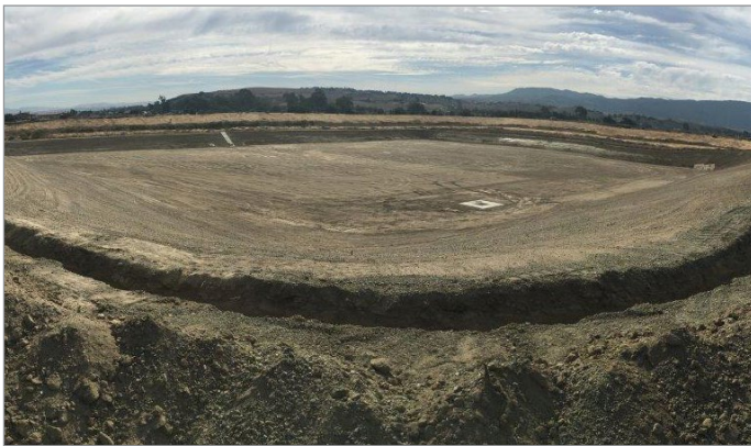
Site ready for installation of liner
