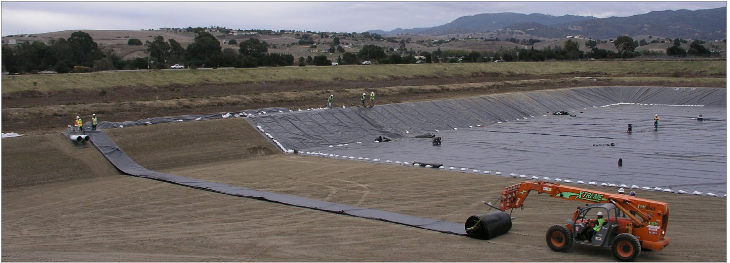
AquaMaster 45L being installed in large panels
